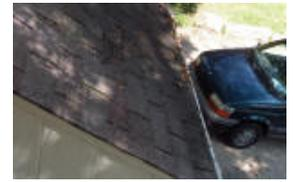
The near constant stream of water through the basement foundation was in part fed by poorly installed and maintained gutters. Note how roofing material covers most of the gutter guard – which Kathy Fountain tried to convince me was a new popular technique. (Click to enlarge)
